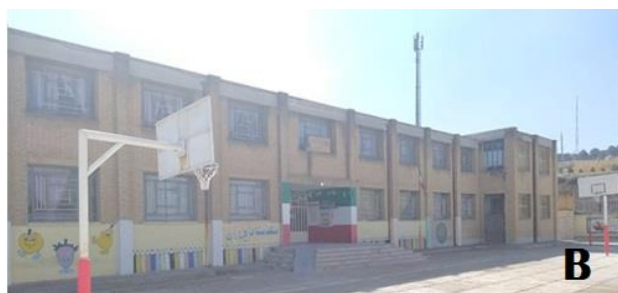
Fig. 1. A: The modeled view of the building in Design Builder software; B: The current state of the Ehsan School building
