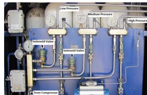
Figure 2. A Schematic diagram of a priority panel for a CNG refueling station
